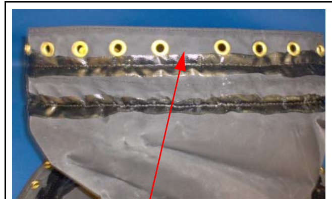
Large gap between grommets and bolt location.
